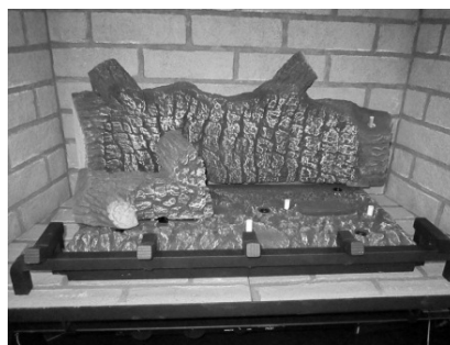
Figure 8: Left Log Installed
