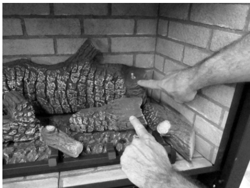
Figure 27: Right Twig Pin
