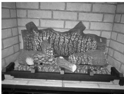
Figure 16: Center Ember Chunk Installed
