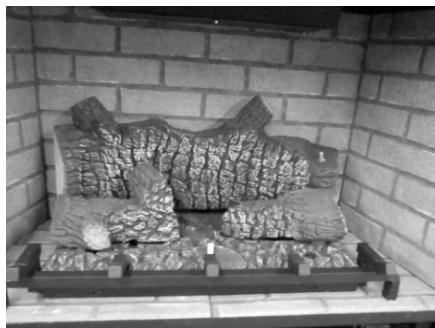
Figure 12: Right Log Installed
